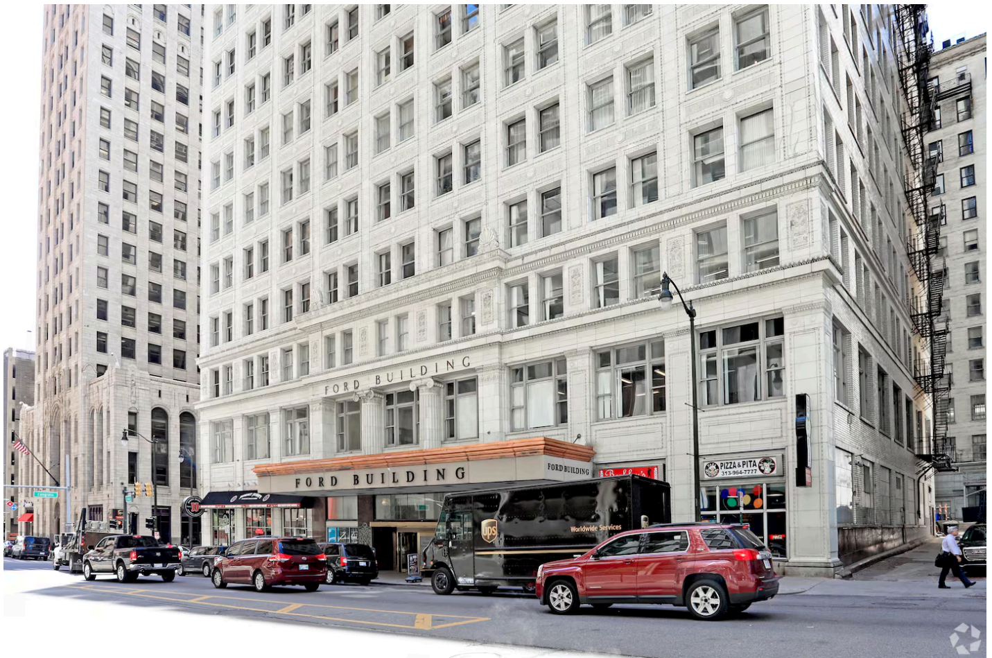
The Ford Building at 615 Griswold St. in downtown Detroit. (CoStar Group Inc.)
